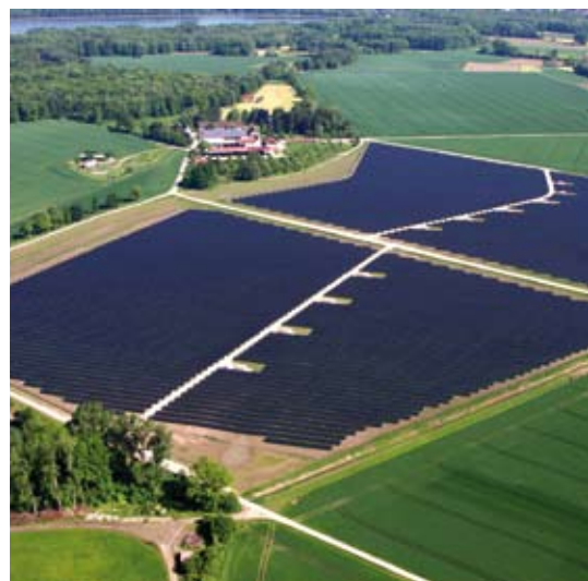
Helmeringen solar park
